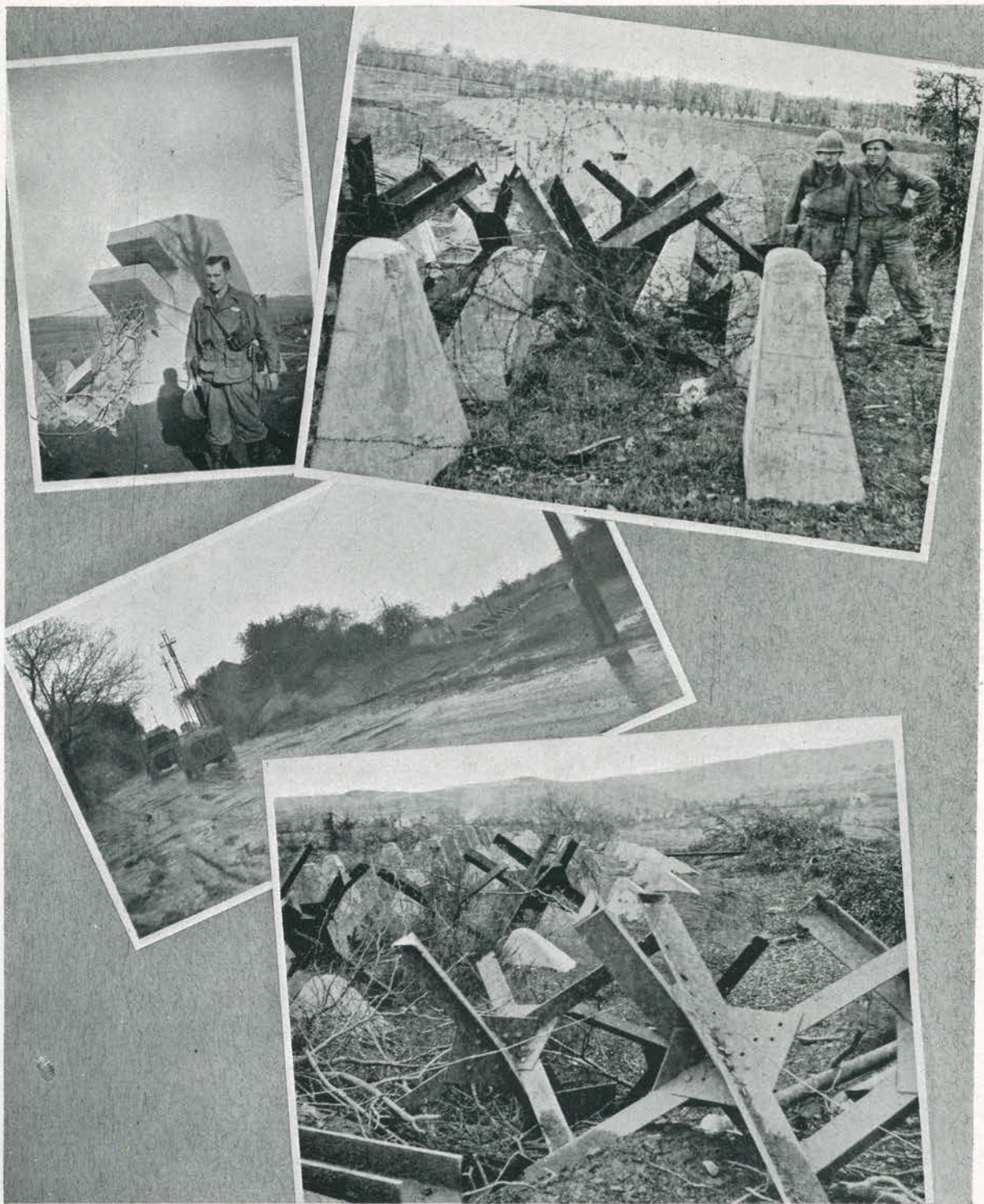
French borders are sown with concrete and steel.
