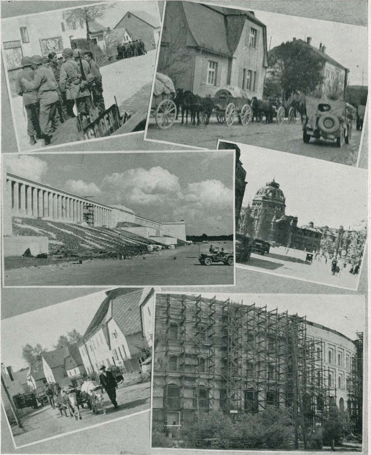
Some of the few buildings still to be seen intact in Nurnberg.
